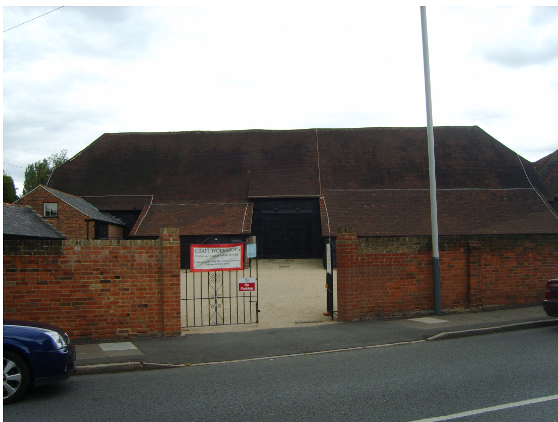
Great Barn viewed from Bury Street
